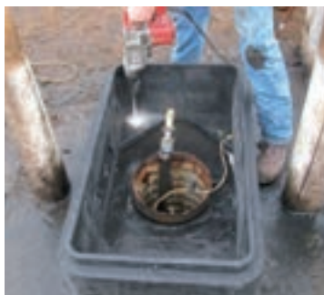
1. Anchor base to concrete
