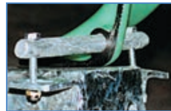
CUTAWAY OF PIN MOUNT
