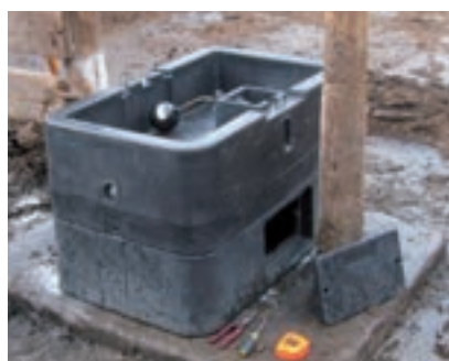
3. Rotate + secure bowl to base
